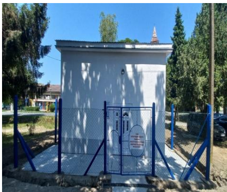
Slika 12. Pumpna stanica Kolut Figure 12. Pumping station Kolut
