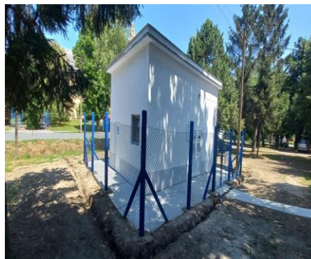
Slika 13. Pumpna stanica Kolut Figure 13. Pumping station Kolut
