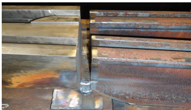
Fig. 3. Preparation for welding the rail base, 3 rd pass
