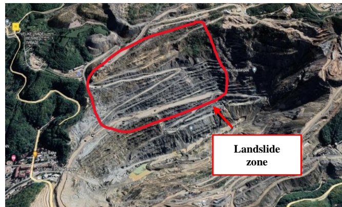
Figure 1. The landslide zone
