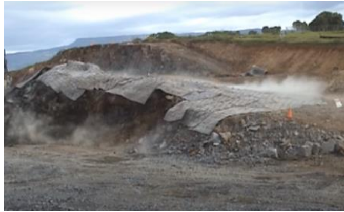
Figure 3. Blasting using the heavy protective covers, initiation of the second order
