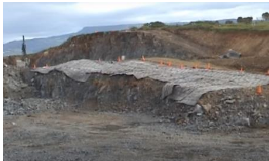
Figure 1. Blasting using the heavy protective covers, before initiation
