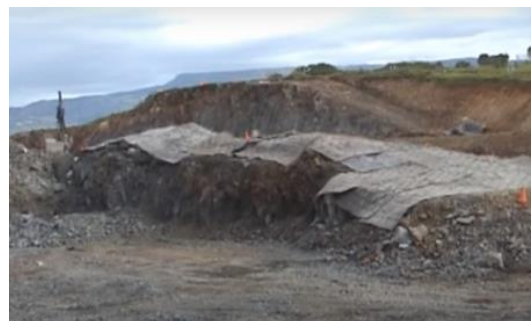
Figure 2. Blasting using the heavy protective covers, initiation of the first order
