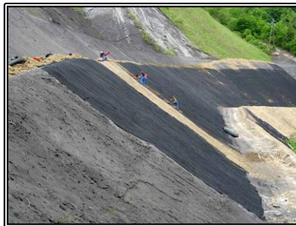
Figure 1 Representation of covering the slope of the landfill with a geogrid
