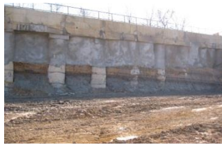
Figure 1. Appearance of the retaining wall of the Durutovići cemetery after construction
