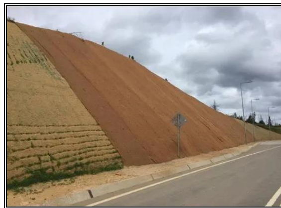
Figure 2. Coconut Geogrid
