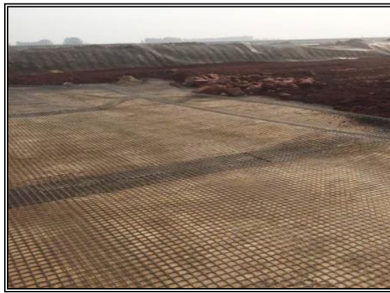
Figure 1. Setting up the geogrid
