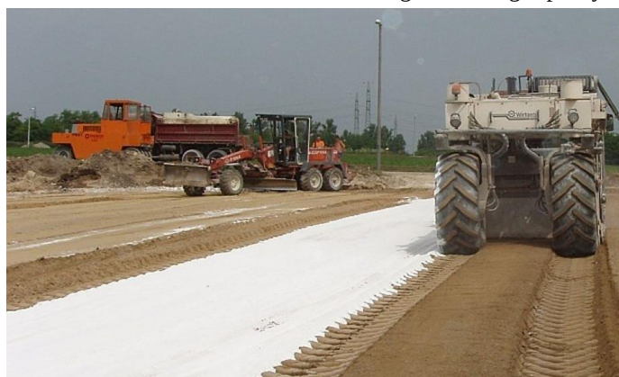
Figure 3. The process of stabilizing the base soil with lime in the field [2]
