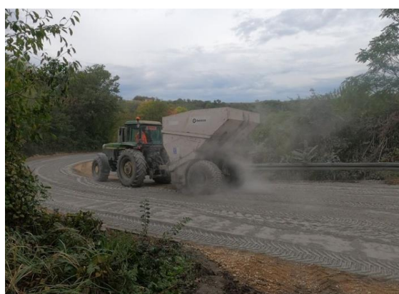
Figure 2. The process of stabilizing the base soil with cement in the field [2]
