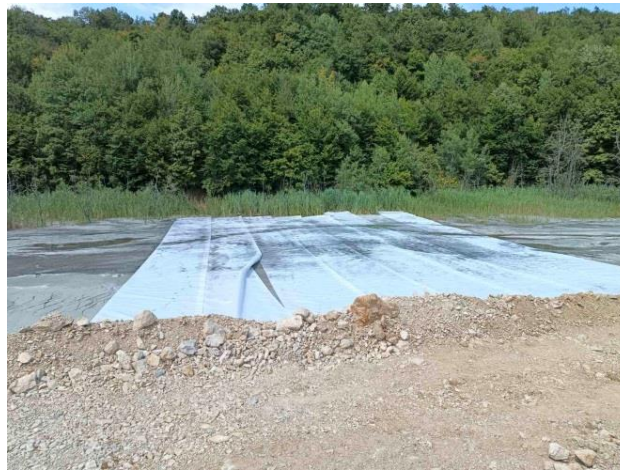
Figure 2. Laying of the geogrid membrane
