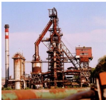
Figure 1. Steel rozonda in blast furnaces (5)
