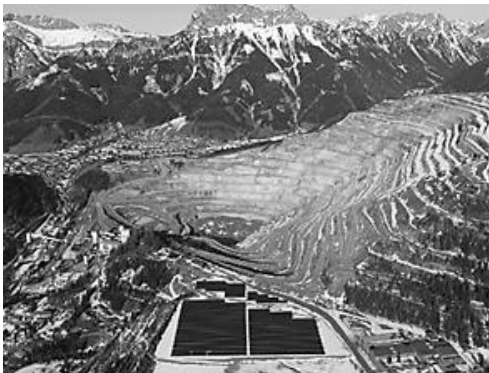
e) solar power plant, Erzberg, Austria [7]
