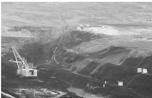
Figure 4, Repeated sliding of disposed material and breakage of coal floors, 2007. [1]
