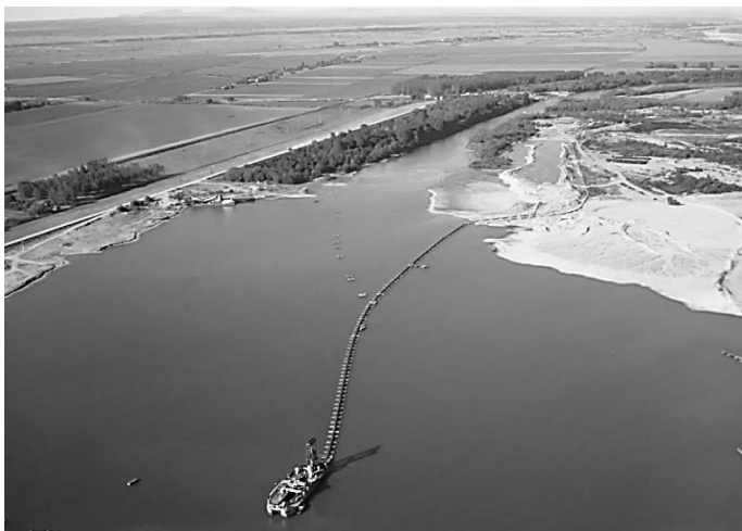
Figure 1, Exploitation system when working on gravel: excavator - pipeline – place of discharge
