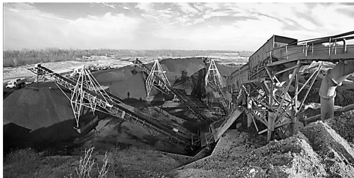
Figure 4, EHS III dewatering and classification plant
