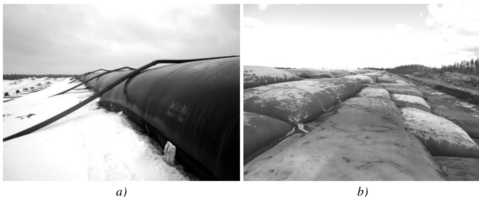
Figure 3, a) The dewatering solution at Talvivaara during winter b) Completed dewatering field with fifth tube layer
