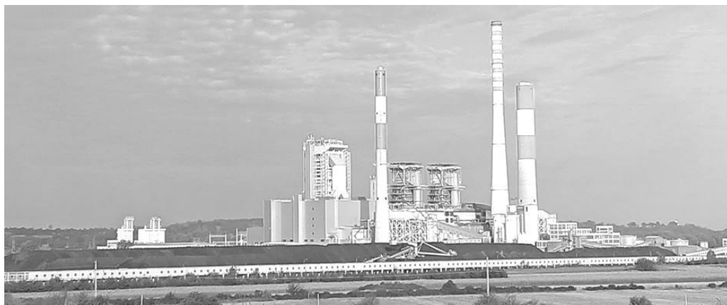
Figure 1, Thermal power plants B1, B2 and B3
