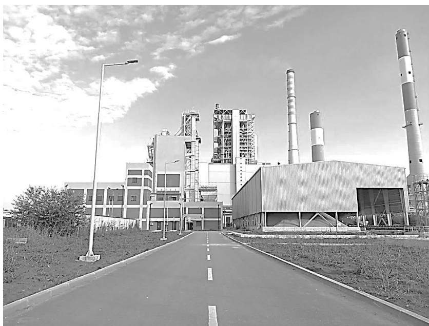
Figure 2, Thermal power plant B3
