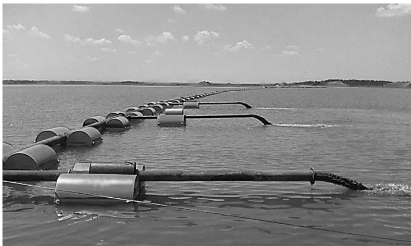
Figure 2, Discharge pipeline on pontoon supports showing the discharge of hydraulic mixture in operation (Photo by Goran Đotunović)
