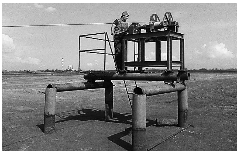
Figure 4, Installed position of the winch at the landfill (Photo by Goran Đotunović)
