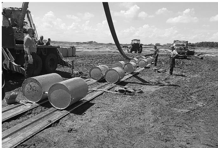
Figure 3, Installation of the discharge pipeline on pontoon supports (Photo by Goran Đotunović)
