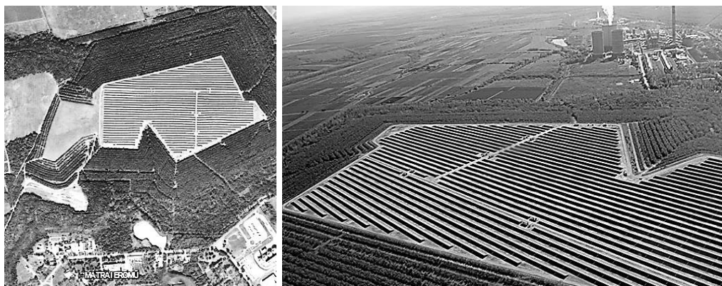
Figure 1, PV solar power plant at the thermogenic waste landfill in TPP Matra
