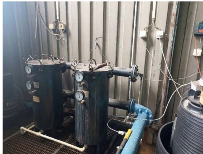
Figure 3. Device for removing iron and adjusting the pH value of returning water in DHP "Krivi Vir" in Niš
