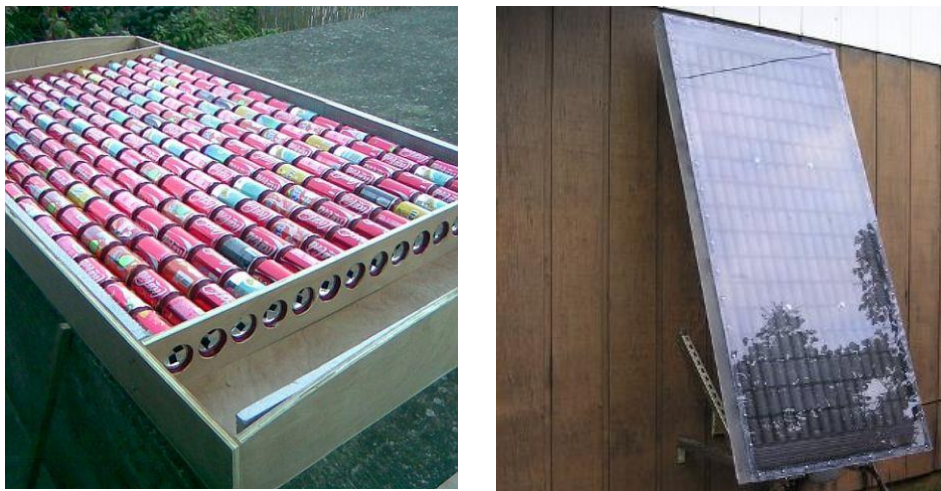
Picture 4. Construction and installation of the solar air collector
