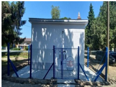
Slika 10. Pumpna stanica Kolut Figure 10. Pumping station Kolut
