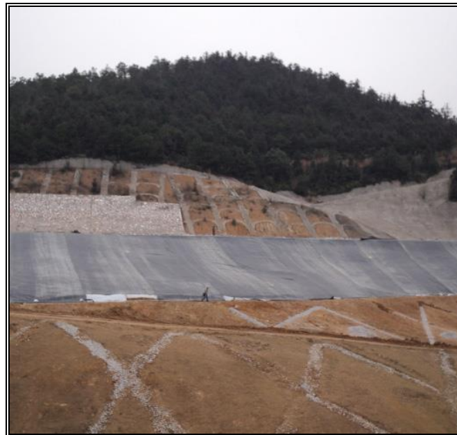
Figure 1. Presentation of covering (covering) the slope of the landfill with a geogrid
