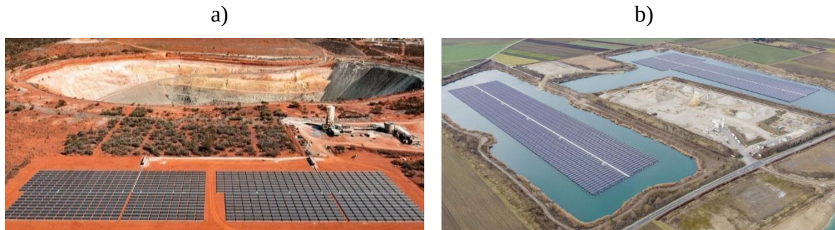
Figure 2. a) The Carosue Dam solar plant in mine (Australia) [11]
