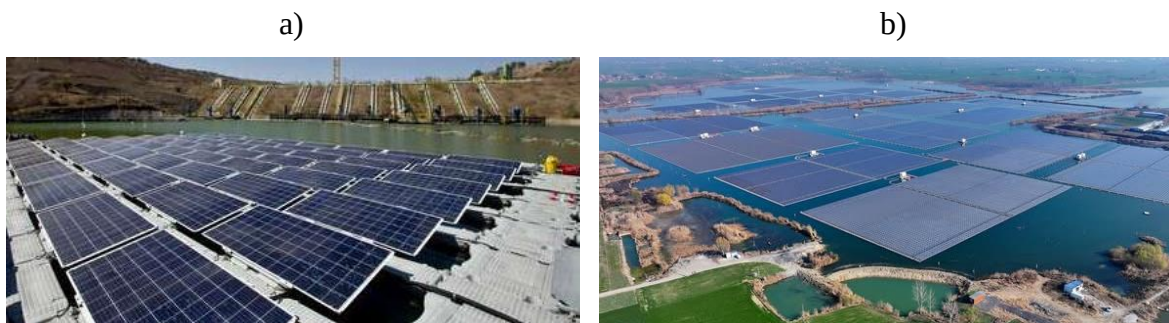
Figure 3. a) Floated solar panels in a pond of “Los Bronces” mining plant (Chile) [13]
