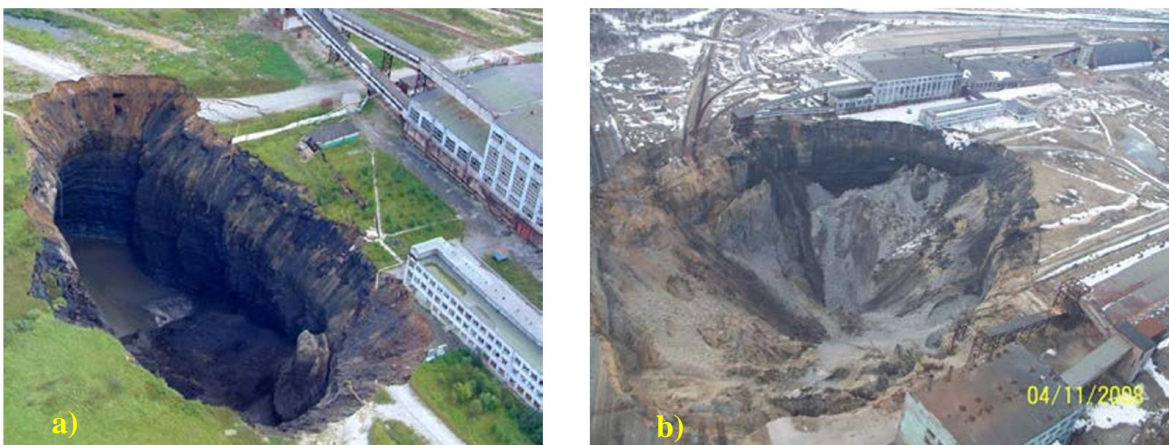
Figure 1. Sinkholes above Berezniki potash mine, Russia: a) June 2007 and b) November 2008 (source: Itar-Tass news agency and ru.wikipedia.org).
