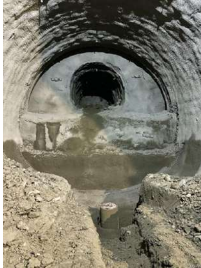
Fig. 4. Pilot tunnel within the excavation profile of the station tunnel (Source: IGT Geotechnik und Tunnelbau).
