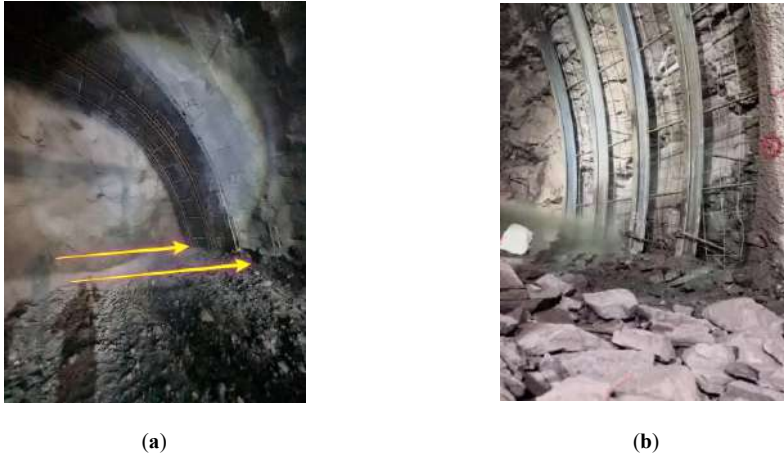
Fig. 2. (a) Primary support without anchors and propiate temporary foundations; (b) Installing multiple steel ribs in the stable ground with no stiff support on the ground.
