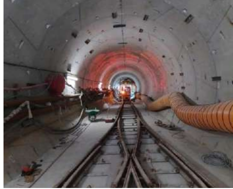
Fig 13. Installation of California switches and final arrangement for TBM regular mining activities.
