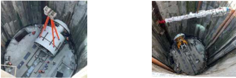
Fig 5. Assembly of the TBM in the shaft.
