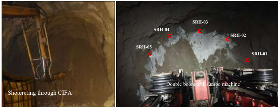
Fig. 10. (a) Application of normal shotcrete and SFRS layer-wise on tunnel face, crown, and side walls; (b) Drilling of stress relief holes (SRH) at the face using a double boom drill jumbo.
