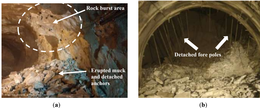
Fig. 9. (a) Rock spalling resulted in detachment of shotcrete and rock anchors around RD \pm 5284 m; (b) Fore poles detached and hanged after multiple episodes of rock bursts at the face and crown around RD \pm 5352 m.
