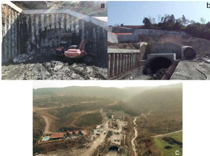
Fig. 12. T1 Tunnel portal construction stages (a: completion of bored pile construction, b: cut-and - cover construction and backfilling stage, c: T1 Tunnel portal completed status).
