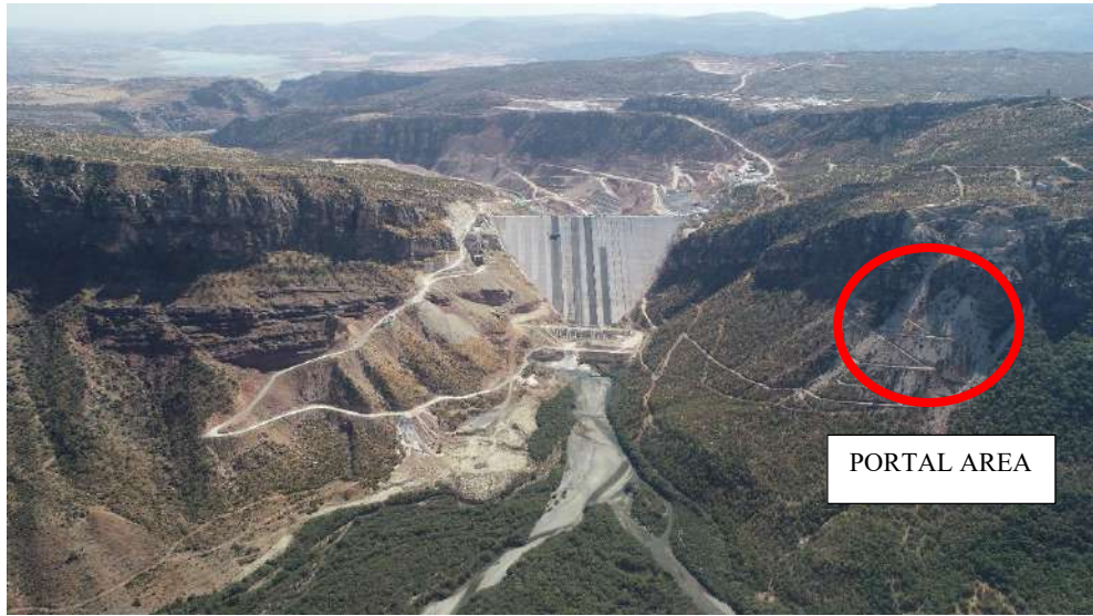
Fig. 2. General view of the portal area.
