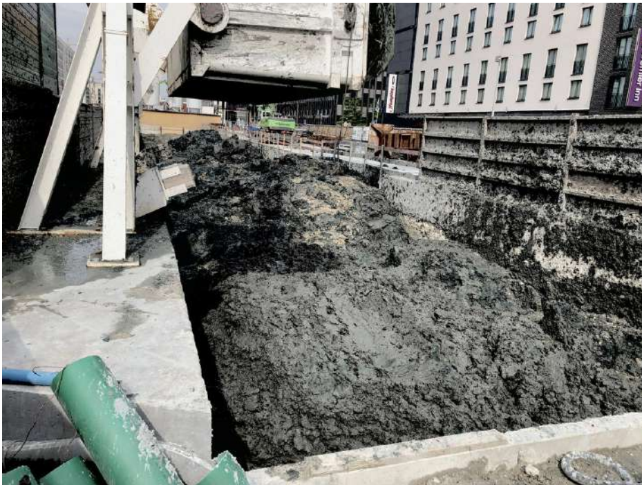
Fig. 12. Conditioned Frankfurt Clay at station surface, June 2020.
