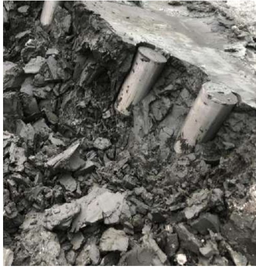
Fig. 9. Frankfurt Clay at Güterplatz, freshly hand-excavated
