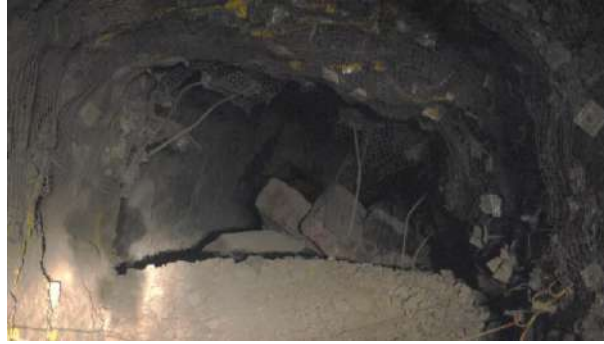
Fig. 6. Blocky metasandstone on extraction level. Block falls observed from hanging wall of unsupported stope.
