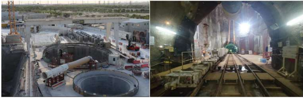
Fig. 5. Photo of the logistics and drop shaft during TBM operations.
