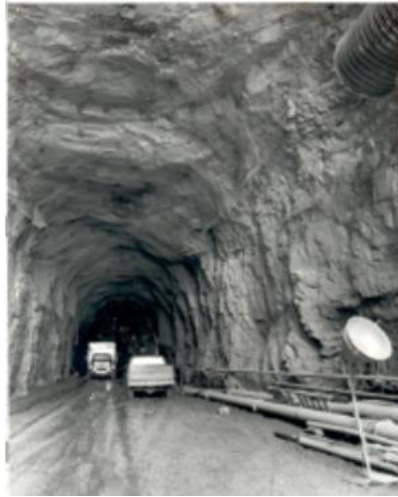
Fig. 9. View of discharge tunnel.
