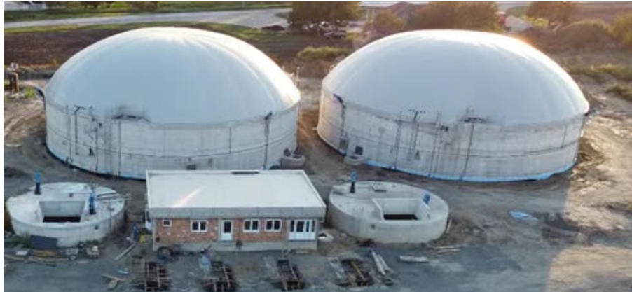
Fig. 2. Circular concrete digester
